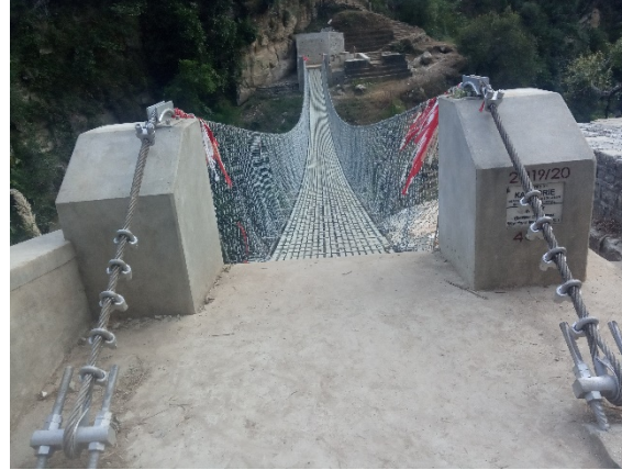
Picture 42: Suspended Bridge
