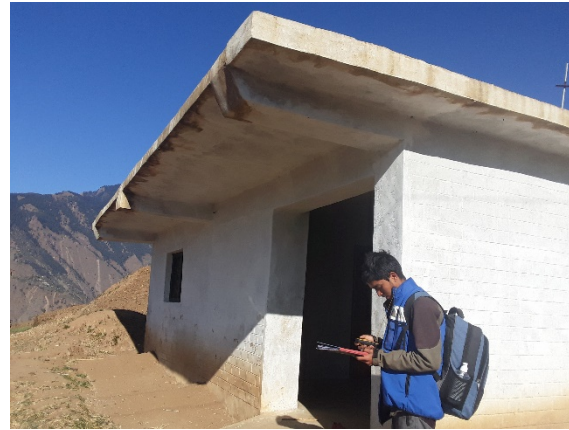
Picture 34: Taking GPS point of Public Buildings
