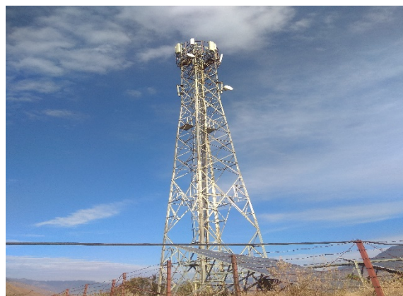
Picture 8: Telecom tower, Manma
