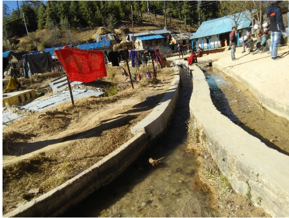
Picture 41: Irrigation Canal
