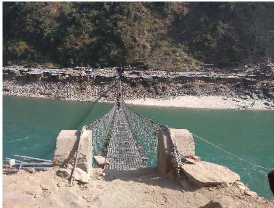
Picture 43: Suspended Bridge
